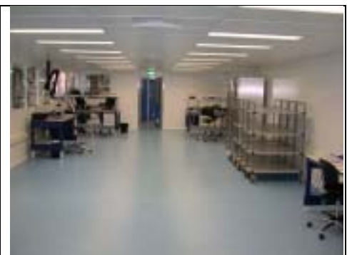
The Clean-room for secure and high quality repair of the electronics or controller.
